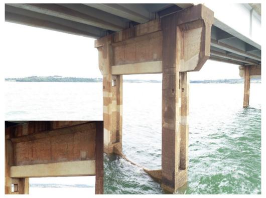
Figure 8. Crossbeam 11 with cracks
