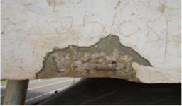
a) Longitudinal beam 3, on overhang 3, with crumbling concrete and exposed reinforcement
