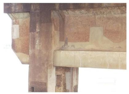
Figure 9. Pillar of support 21 with cracks on the repair.
