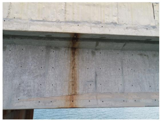
**Figure 10.** Span 12 of the longitudinal beam 2, with signs of water infiltration. It was possible to note the absence of an extension tube on the drainpipe.
