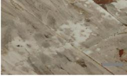
b) Deck slab with crack showing efflorescence
