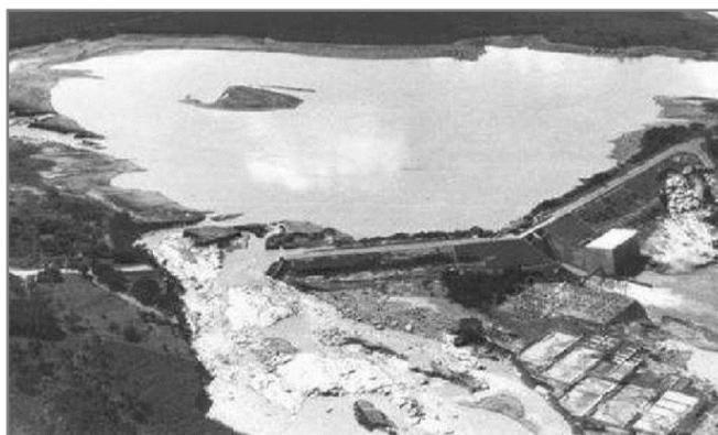
**Figure 2.** Rupture of dam Armando Sales de Oliveira after the cascade overtopping on 01/21/1977 (Saliba, 2009).
