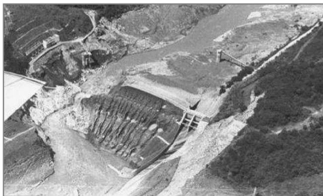
**Figure 1.** Rupture by overtopping of the Euclides da Cunha dam (Saliba, 2009).
