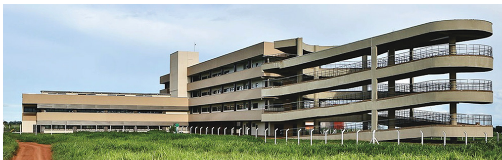
Figure 1 - Side view of the building (Mesquita, 2019).
