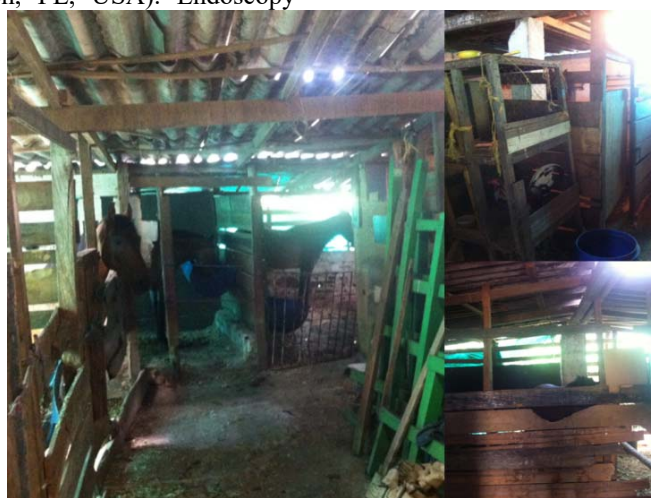
Figure 1. Inadequate ventilation in one of the farms showing accumulation of debris and presence of other animal species stabled with the horses.
