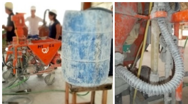
Figure 6 - Mortar water dosage - construction work C
