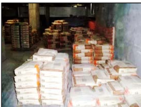
Figure 7 - Stock of the dry-mix mortar in the basement
