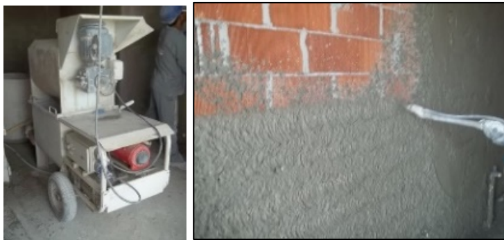
Figure 4 - Sprayer Equipment BETOMAQ - construction work C
