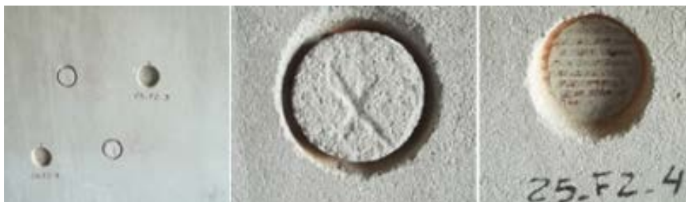
Figure 9 - Tensile bond test site
