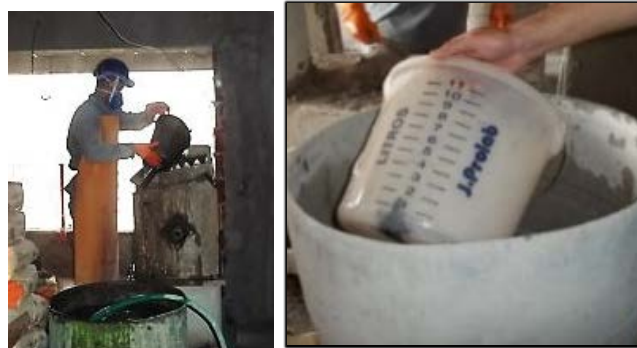
Figure 5 - Water dosage in the mortar - construction work B
