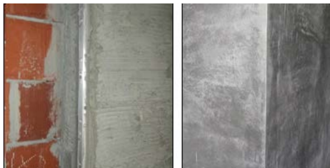
Figure 10 - Use of corner-beds in corner and edge places
