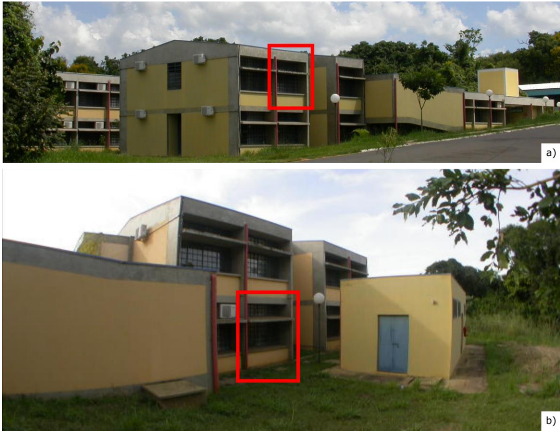
Figure 2 - (a) Front facade (NNE) of the DESIGN building, highlighting the position of the room to be modeling; in the background is the front facade of the DAUP building; e (b) rear facade (SSO) of the DAUP building, highlighting the position of the room to be modeling - users of the two ground floor rooms located behind the electric power cabin did not respond to the questionnaires, since they are out of the general pattern, with a large obstruction facing the windows
