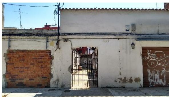
Figure 2 - Property to be demolished at Carrer Ramon Turró
