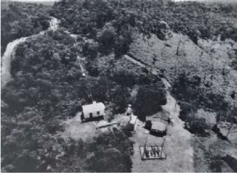
Figure 2 - Aerial photo of the Bagagem SHP
