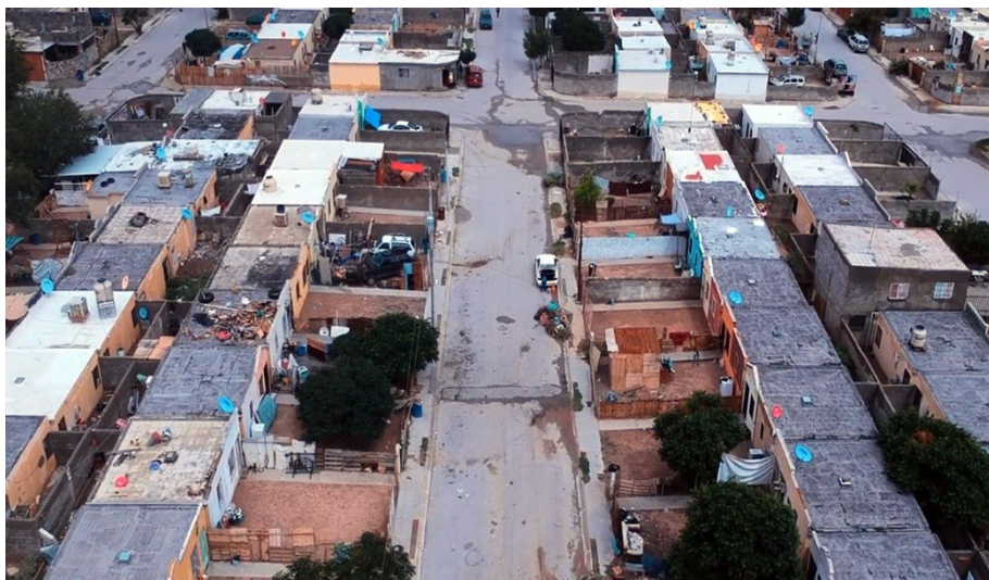
Figure 4 – Senderos de San Isidro housing estate
