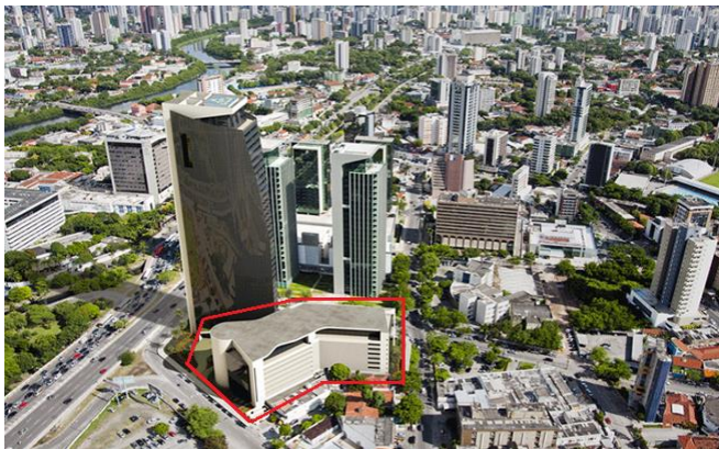
FIGURE 1. Location of the Charles Darwin Building's Parking Garage, Rio Ave Empreendimentos, in Recife, PE, Brazil.
