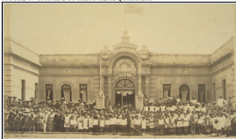
FIGURE 1 – FACADE OF A.E.A. HEADQUARTERS
