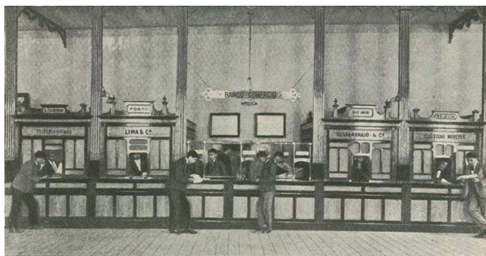
Figure 18 - Commercial offices in Escola Prática Comercial Raul Dória .
