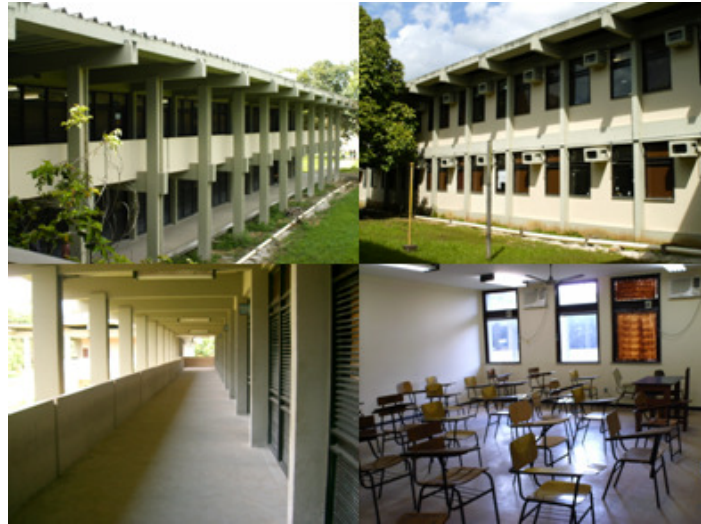
Fig. 1. Pictures of the building. Clockwise from top right: external elevation with glass windows, classroom, corridor, and external wall with corridor.
