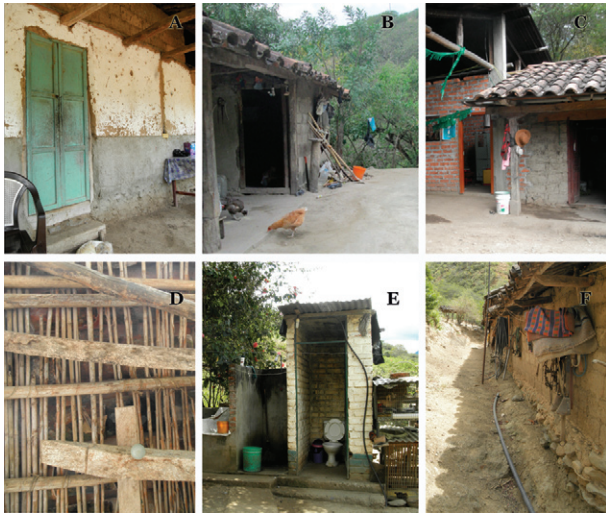
Fig. 1: positive deviants have implemented different solutions to deter the natural decay of their houses and reorganise their living environments. Improvements applied to traditional adobe structures include: cement plastering (A), cement floors in the porch area (B), partial additions constructed with bricks (C), carrizo ceiling and chahuarquero beams (D), latrines and water tanks (E) and rock foundations (F).
