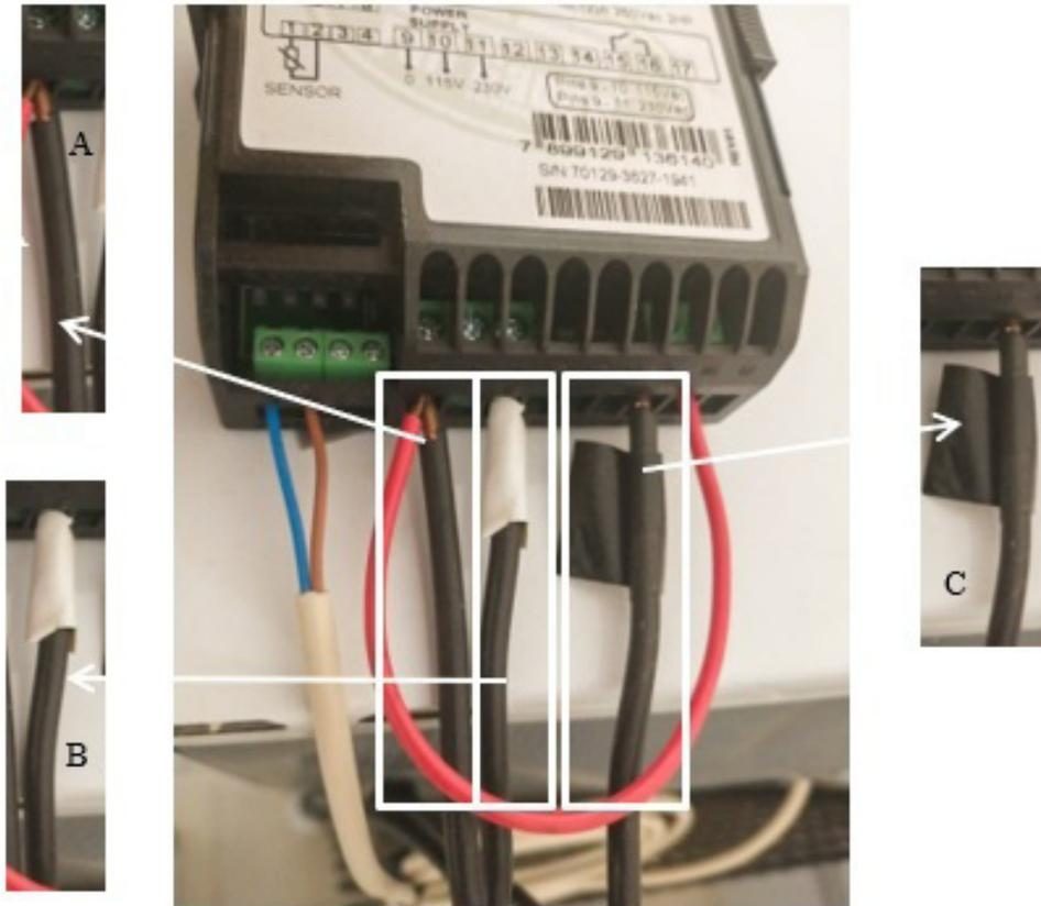
**Figure 5.** Red wire (jumper) connecting terminal 9 to 16: (A), 220V phase for the temperature controller; (B) wire from neutral to the controller; (C) 220V phase wire for the compressor.
