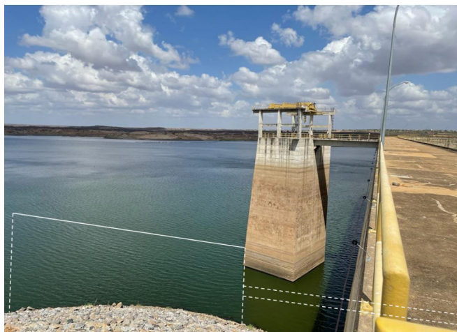
Figure 4. Water intake tower of Castanhão reservoir. A sketch of the control volume used in the numerical simulations of the flow approaching and inside the water intake pipeline is also indicated.
