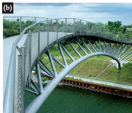
Ripshorster Bridge, Germany
