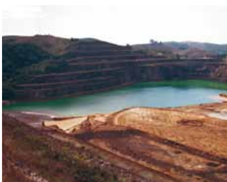
Figure 5 Osamu Utsumi pit partially filled with water, pH=3,5 on the left and “waste dump” 4 on the right. The lake in bottom of the “waste dump” 4 is formed by water drained from it, pH = 2,5. The water from the “waste dump” is pumped to the pit and then to an active water treatment system.
