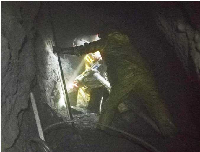
Figure 1 - Rock drilling (downwards). Source: Universidad Adolfo Ibañez
