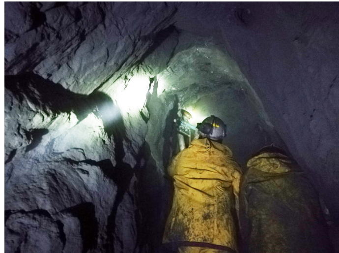
Figure 2 - Rock drilling (upwards). Source: Universidad Adolfo Ibañez
