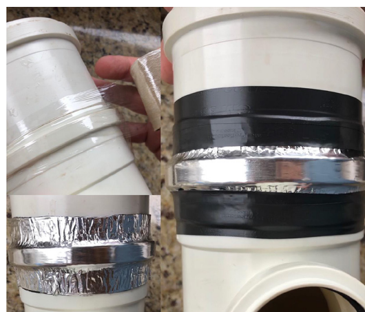
Figure 8 – Sealing procedure in the junction.
