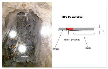
Figure 7 - Blast 2: drilling and charging configuration.
