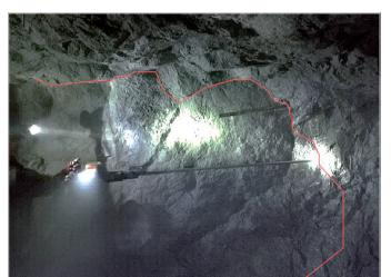
Figure 3 - Result of blasting at the Mina La Palmera, showing the overbreak profile.
