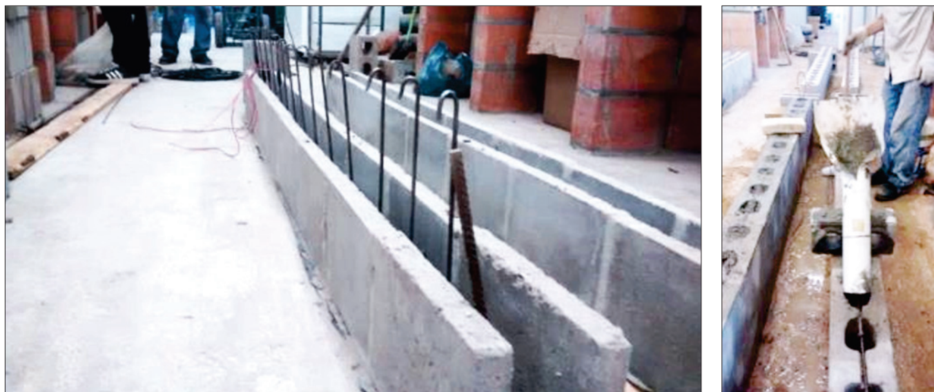
Figure 9 First course with stirrups (left) and grouting (right)
