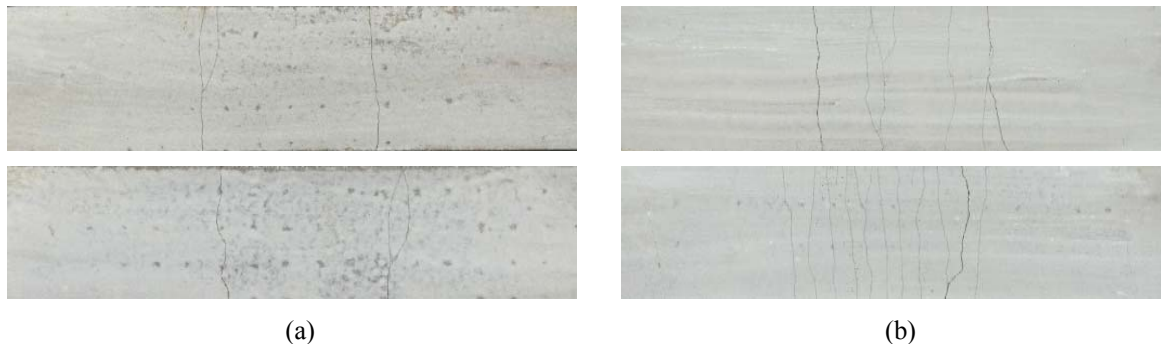
Figure 6: Typical cracking patterns For: (a) R2%_50 composite and (b) R4%_50 composite.
