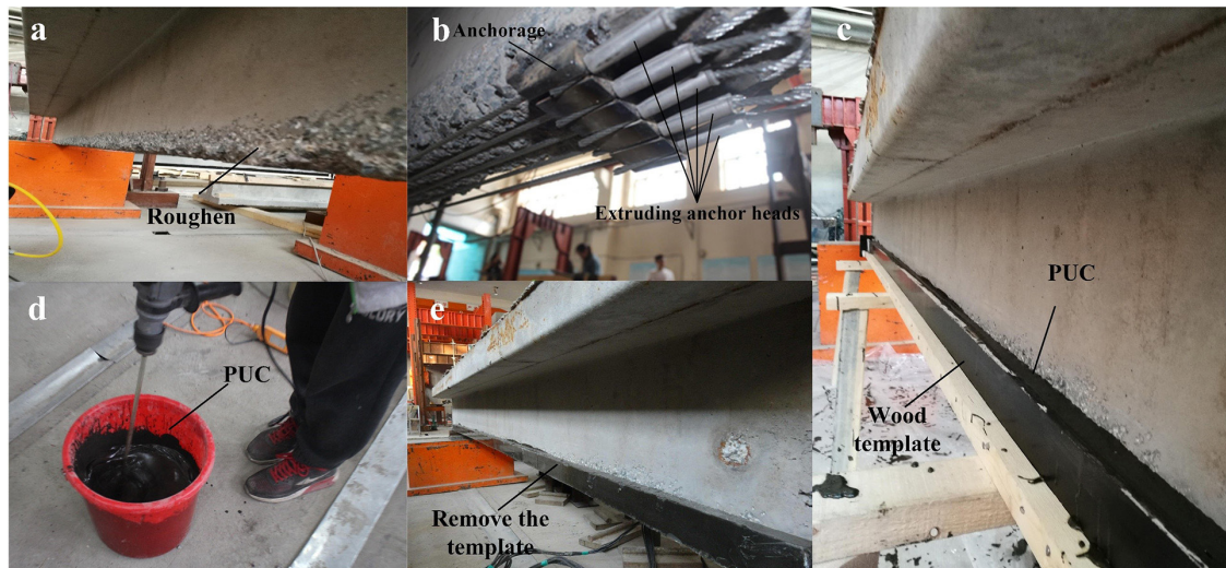
Figure 4: Operation procedure of PSWR-PUC reinforced beams: (a) concrete surface preparation, (b) tensioning and anchoring the prestressed wire rope, (c) fixing wood template and casting the PUC material, (d) Mixing and stirring the PUC material, (e) Removing the wood template.
