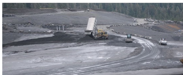
Figure 1. Filtered dry stack tailings at Greens Creek mine, Alaska (Wilson & Robertson 2015).
