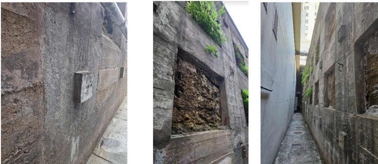
Figure 7. Tieback wall pictures.
