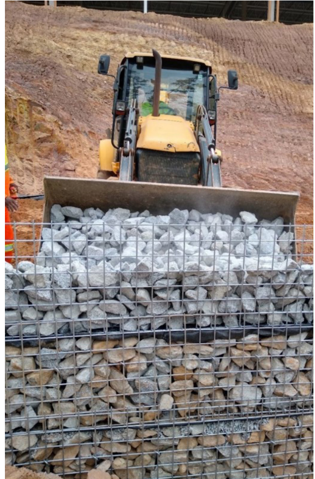
Figure 15. Filling the face modules with small rocks.
