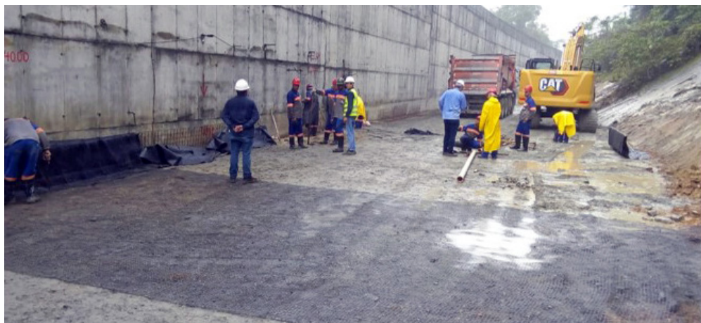
Figure 7. Execution of compacted backfill.
