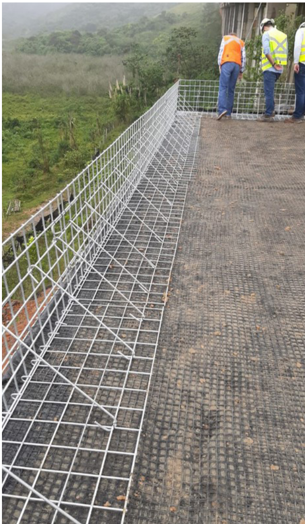
Figure 14. Assembling the face modules.
