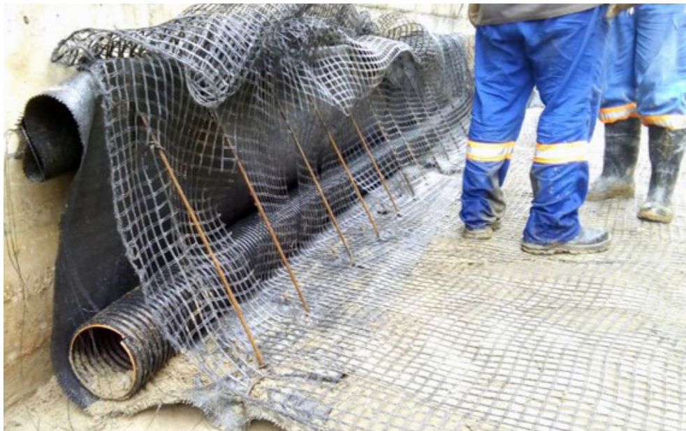
Figure 10. Drainage pipe in the reinforced soil base behind the concrete wall.
