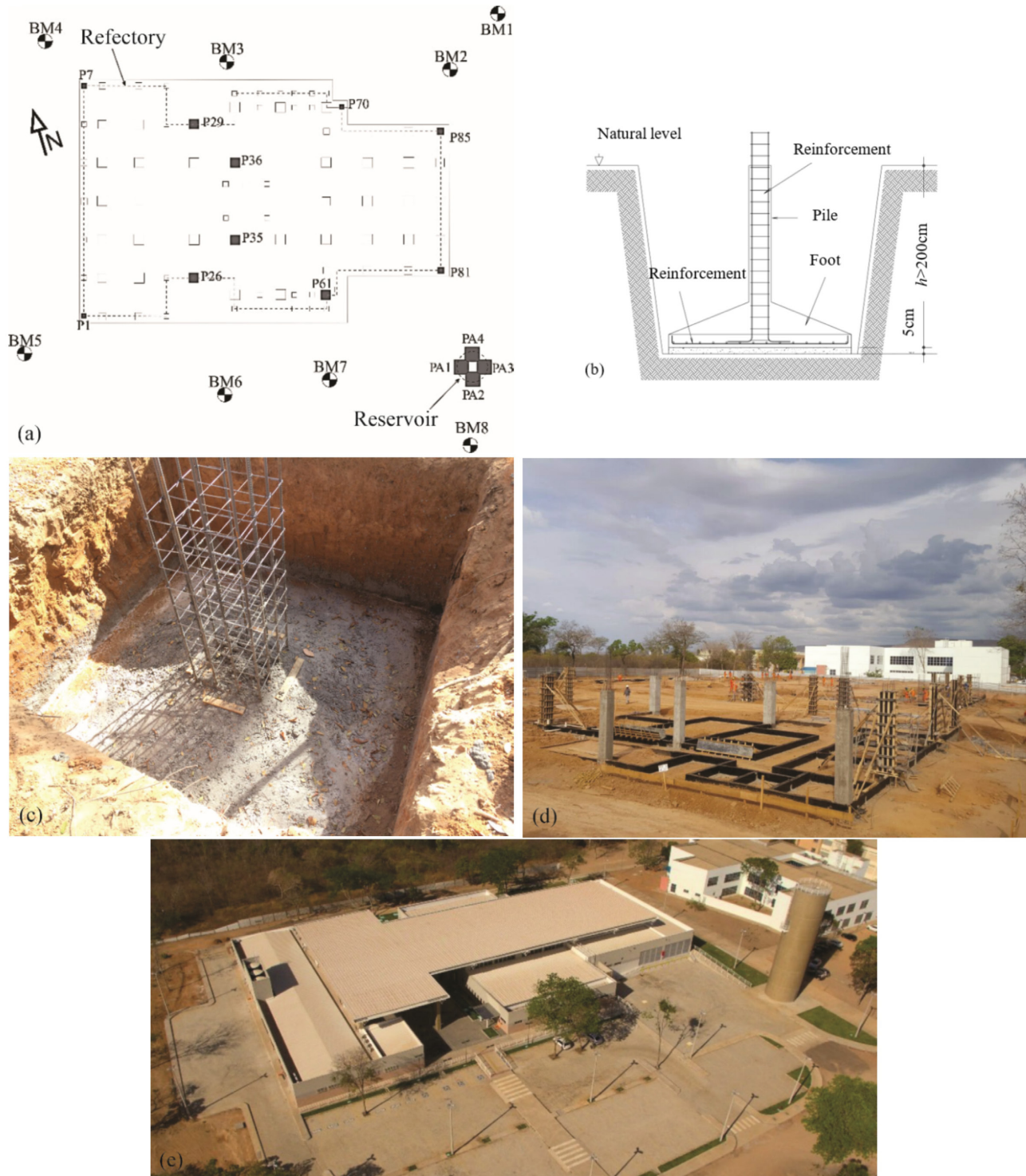
Figure 3. (a) Location of reference points and isolated footings; (b) General support elevation; (c) Isolated footing; (d) Refectory during construction; (e) Buildings after construction.
